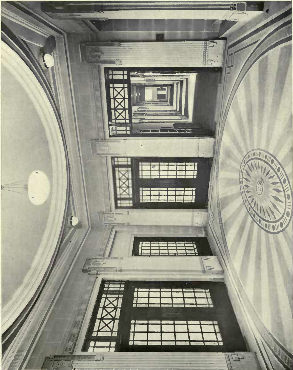
GENERAL ELECTRIC CO., WITTON, BIRMINGHAM : ENTRANCE HALL.
